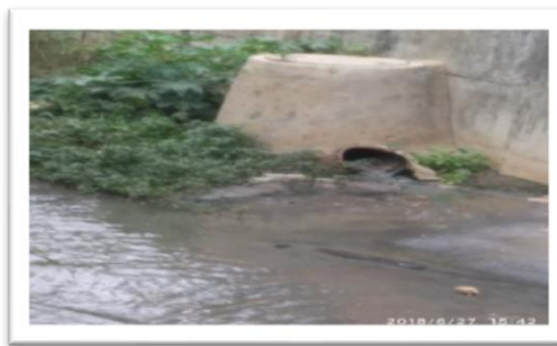
Discharge of sewage into SWD through fractured manhole at Yeshwanthpur, RR Nagar Zone
