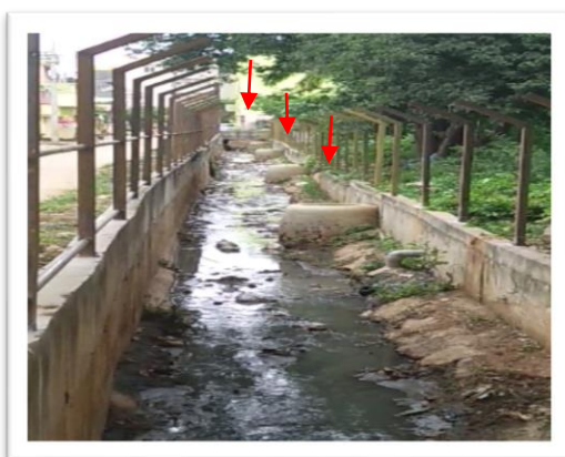
Sewage flowing in the SWDs due to chain of fractured manholes in the drain connecting to Herohalli Lake, Dasarahalli Zone
