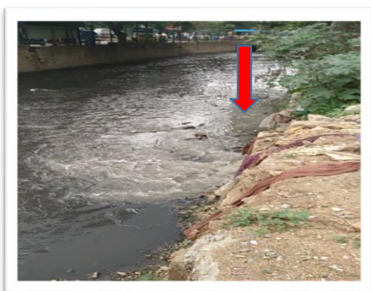
Discharge of sewage into SWD through BWSSB pipeline at Silk Board Junction, Bommanahalli Zone
